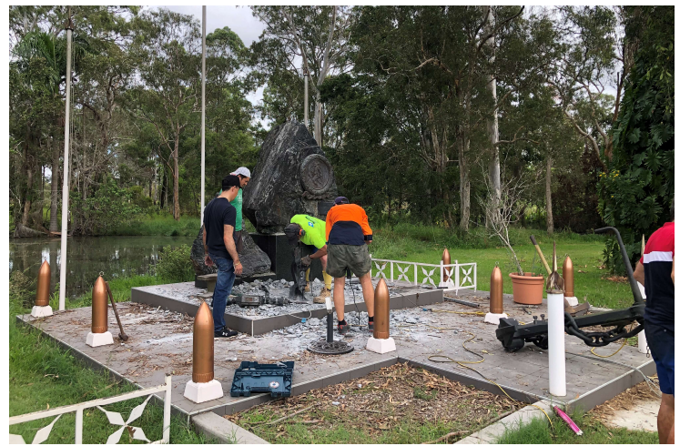
Young volunteers at work preparing for the relocation of the monument.
